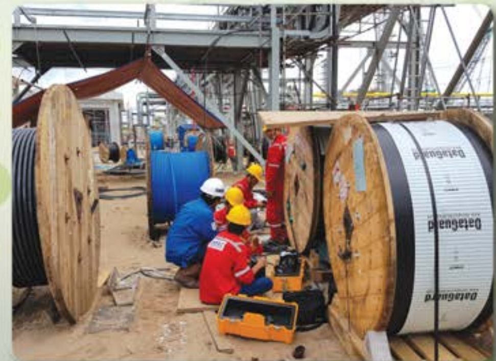
F.O.C – TESTING WORKS
