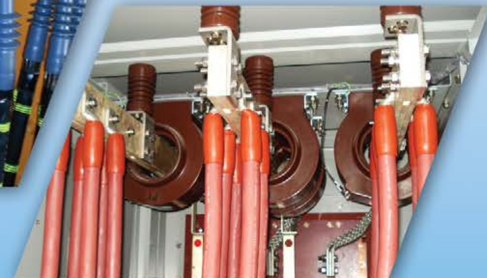
HV – TERMINATION WORKS (22 kVA)
